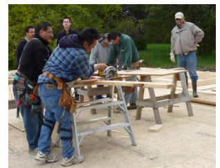
Volunteers hard at work on United Church upgrade project.
