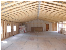
A look inside the United Church hall currently being constructed.
