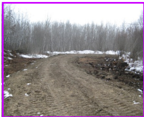
Construction on roadway to camp is now completed
