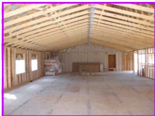
Hall extension on the United Church was completed ahead of schedule
